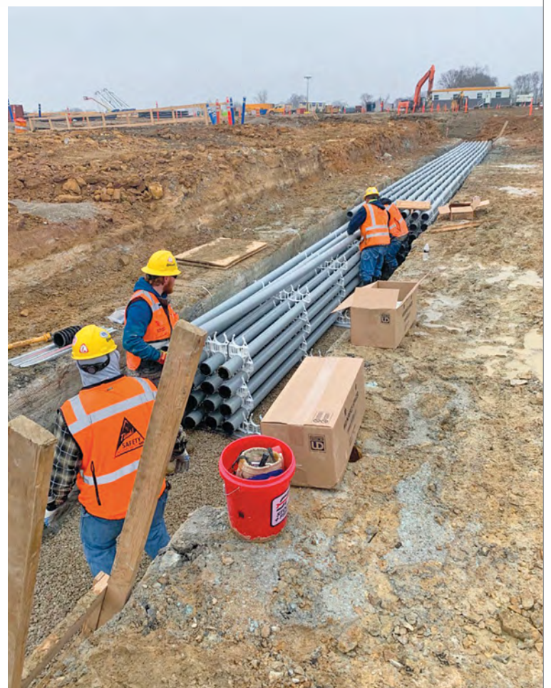
Local 176 members work on the CPV Combined Gas Plant Project.
