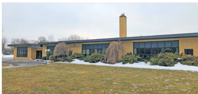
Local 237 completed purchase of a former grade school in Bergholtz, NY, that will serve as its new training facility and union hall.
